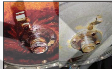
Vessel cover contaminated
